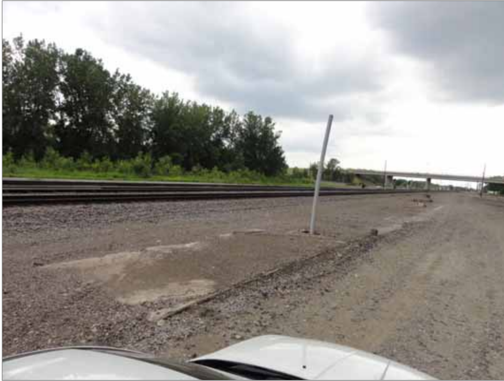
Photo 1: Concrete Slab Foundation
