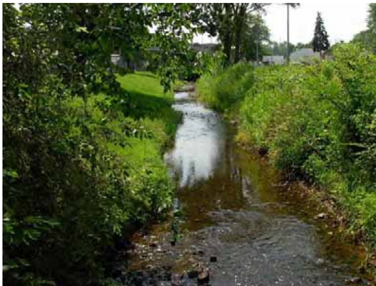
Looking south at Indian Creek channel flowing north within the west end of the Eola Yard, west of Farnsworth Avenue
