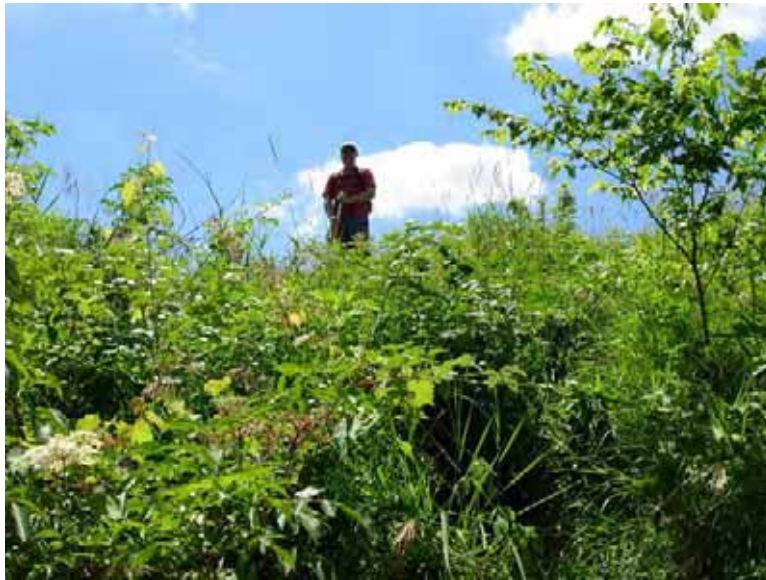
17. Looking from within Pond Creek at a typical bank height of 15-20 to the top of bank.
