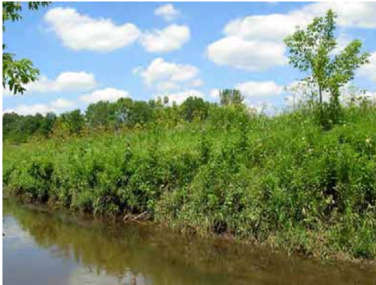
11. Looking at a typical slope along the north bank of Pond Creek, slopes of approximately 1.5:1
